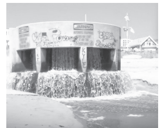
Sea Avenue stormwater outfall, Pt. Pleasant Beach, NJ
