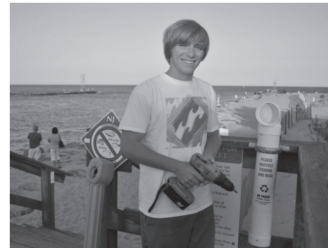
Luke Hayduk installs a fishing line recycling receptacle at Belmar Inlet
