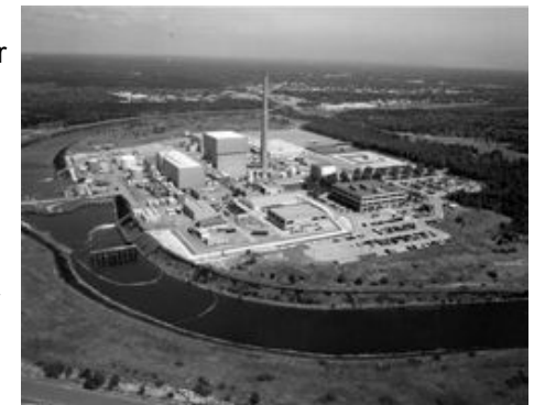
Aerial view of the Oyster Creek Nuclear Generating Station in Lacey Township
